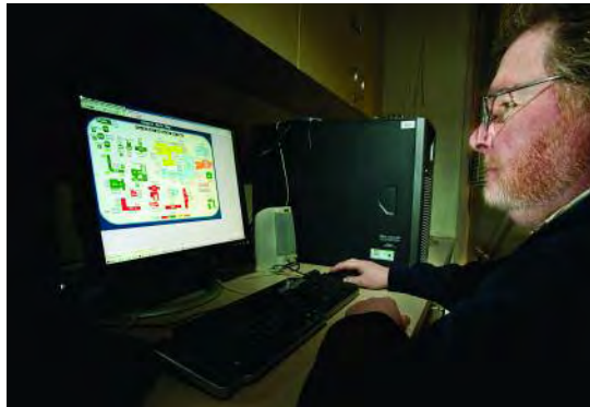
Sophisticated upgrades to the College's computerized energy management system allow service coordinator Bill Brooks (bottom) to monitor 8,000 points on campus and adjust heating and cooling units with the touch of a computer key.
