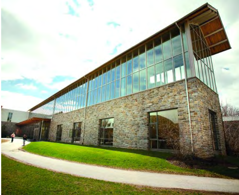
The Committee for Environmental Responsibility pushed to make the Gardner Integrated Athletic Center a green design. The College's first LEED-certified building, it won a gold rating from the U.S. Green Building Council.
