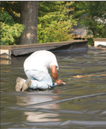
Polyethylene sheeting is installed as a root barrier.
